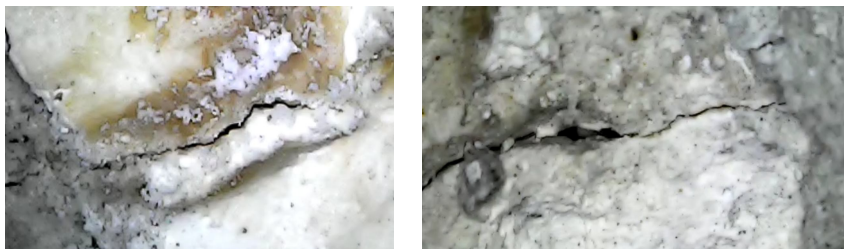
Fig. 8. Cracks in the structure (large scale)
