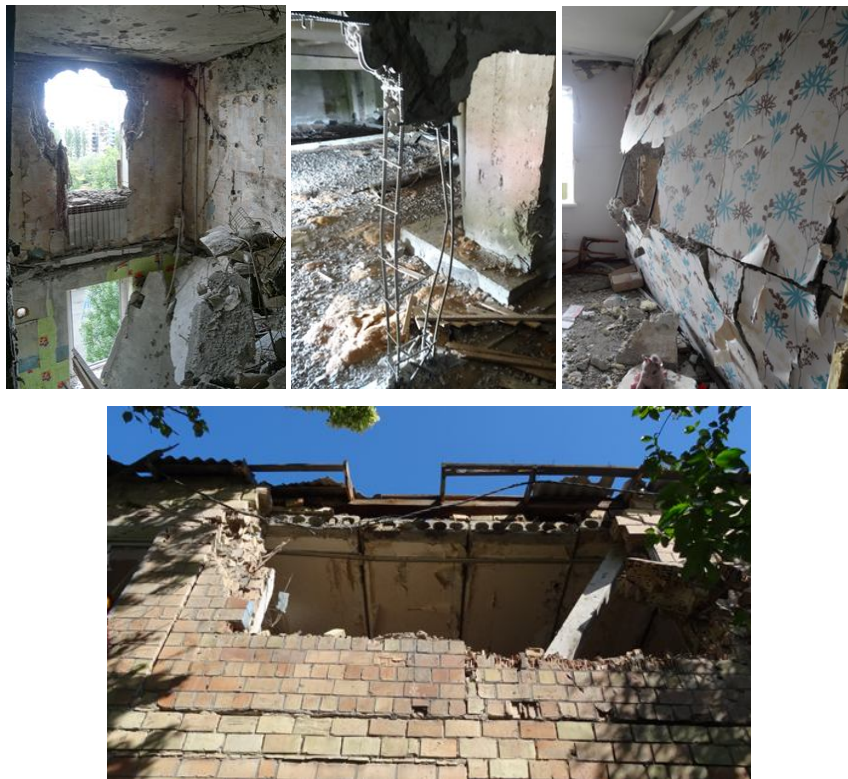
Fig. 4. Damage to structures due to the impact of projectiles from an MLRS, artillery, and tanks
