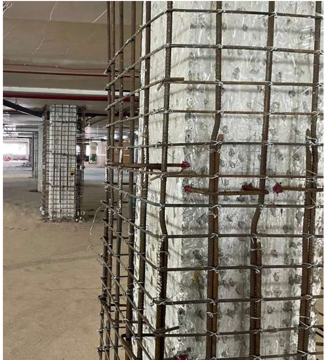
Fig. 1. An example of concrete overlay / jacketing in columns
