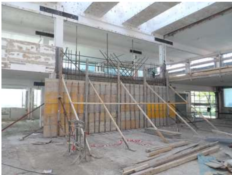
Fig. 2. Example of a shear-in fill wall between columns
